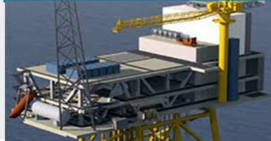
Statoil Valemon, Maintenance & Modification Contract →2016
